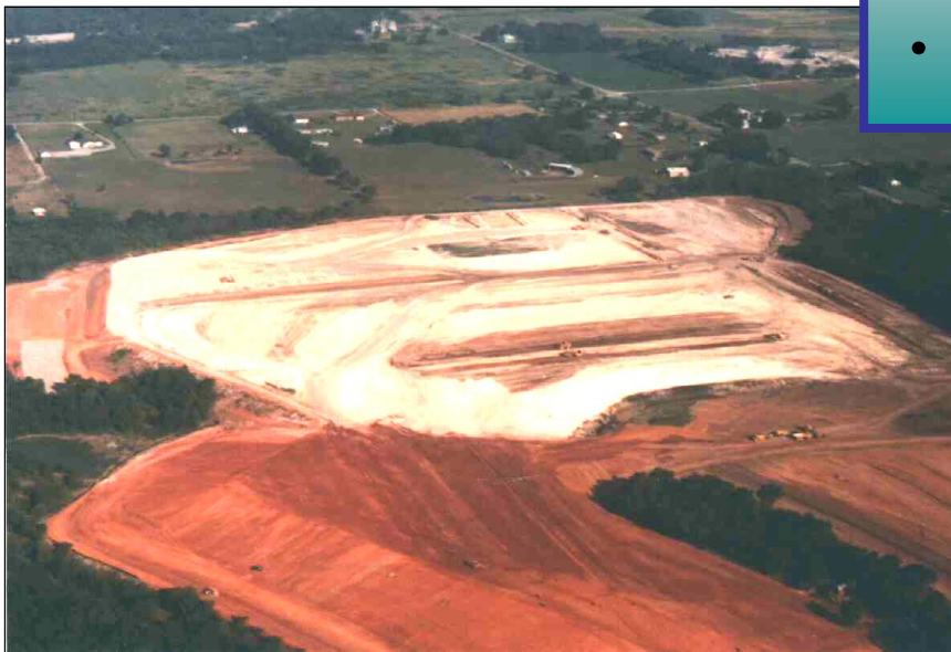
Piles of phospho-gypsum being regraded and covered prior to revegetation.
